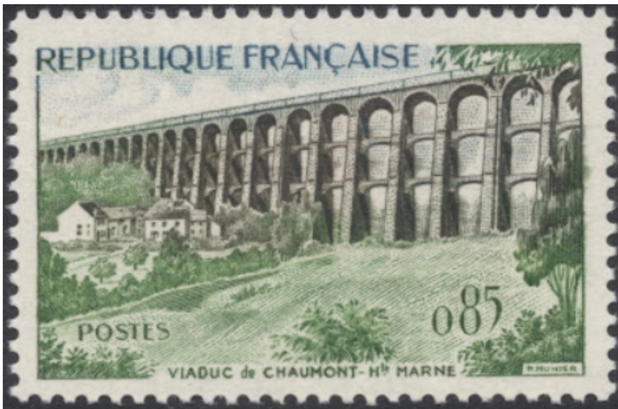
Viaduct Chaumont Haute Marne 1960
